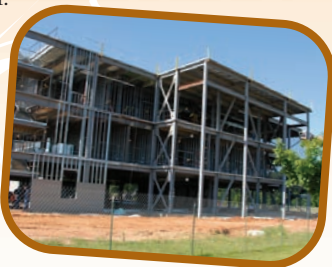
White Hall progress
